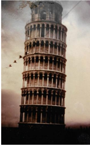
Leaning Tower of Pisa
